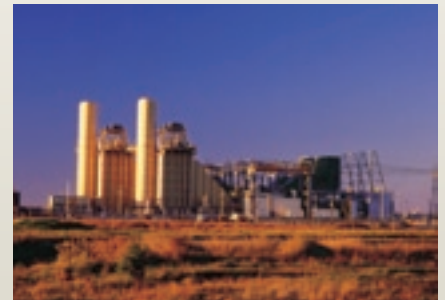
BAYSIDE Canada 1 x KA24-1 MS – 265 MW at 56% net eff. from 100 MW oil fired STPP
