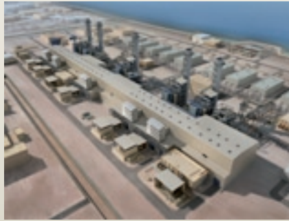
FUJAIRAH F2 UAE 2 x KA26-2 and 1 x KA26-1 – 2000 MW Steam for desalination
