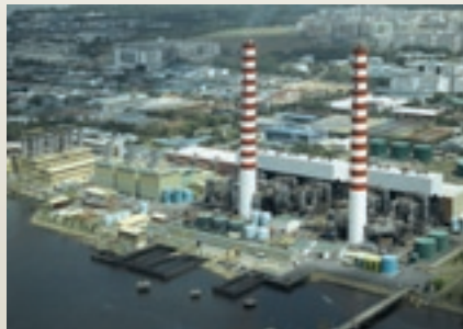
SENOKO Singapore 1 x KA26-1 MS – 360 MW + 2 x KA26-1 MS – 740 MW at 56% net eff. from 3x 120 MW oil fired STPP
