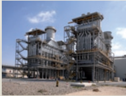
DUBAL PP Ext CCPP22 UEA 1 x KA13E2-2 – 430 MW
