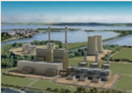
CLAUS C The Netherlands 1 x KA26-3 MS – 1280 MW at 59% net eff. from 640 MW gas fired STPP
