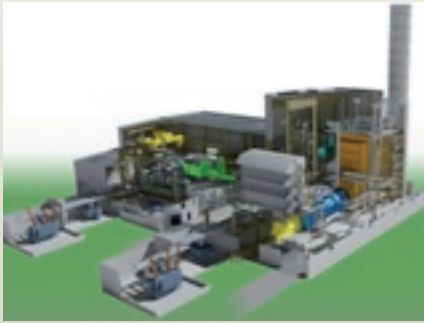
MOSCOW TPP26 Russia 1 x KA26-1 MS – 420 MW District heating
