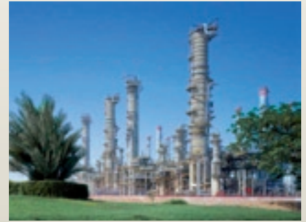
RUWAIS United Arab Emirates 4 x GT13E2 – 500 MW + 8 MIGD* fresh water
