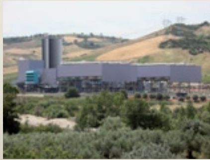
GISSI Italy 2 x KA26-1 SS – 760 MW
