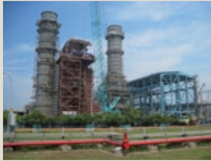
MUARA TAWAR 5 Indonesia 1 x KA13E2-1 – 234 MW (in construction)
