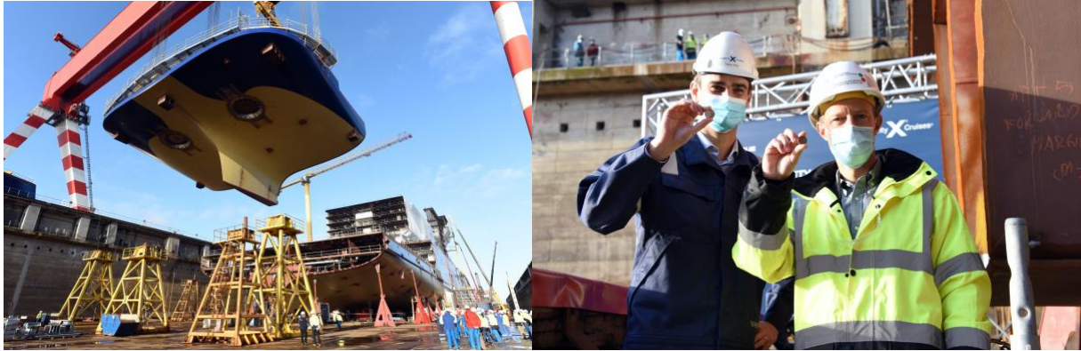
Tobias King, Celebrity Cruises' Edge Series Project Manager, and Sébastien Le Boulluec, Chantiers de l'Atlantique's Edge Series Project Manager, hold the ceremonial "good fortune" coin for Celebrity Beyond as the ship's keel is laid. Celebrity Beyond is the highly-anticipated third ship in the brand's award-winning Edge Series.
