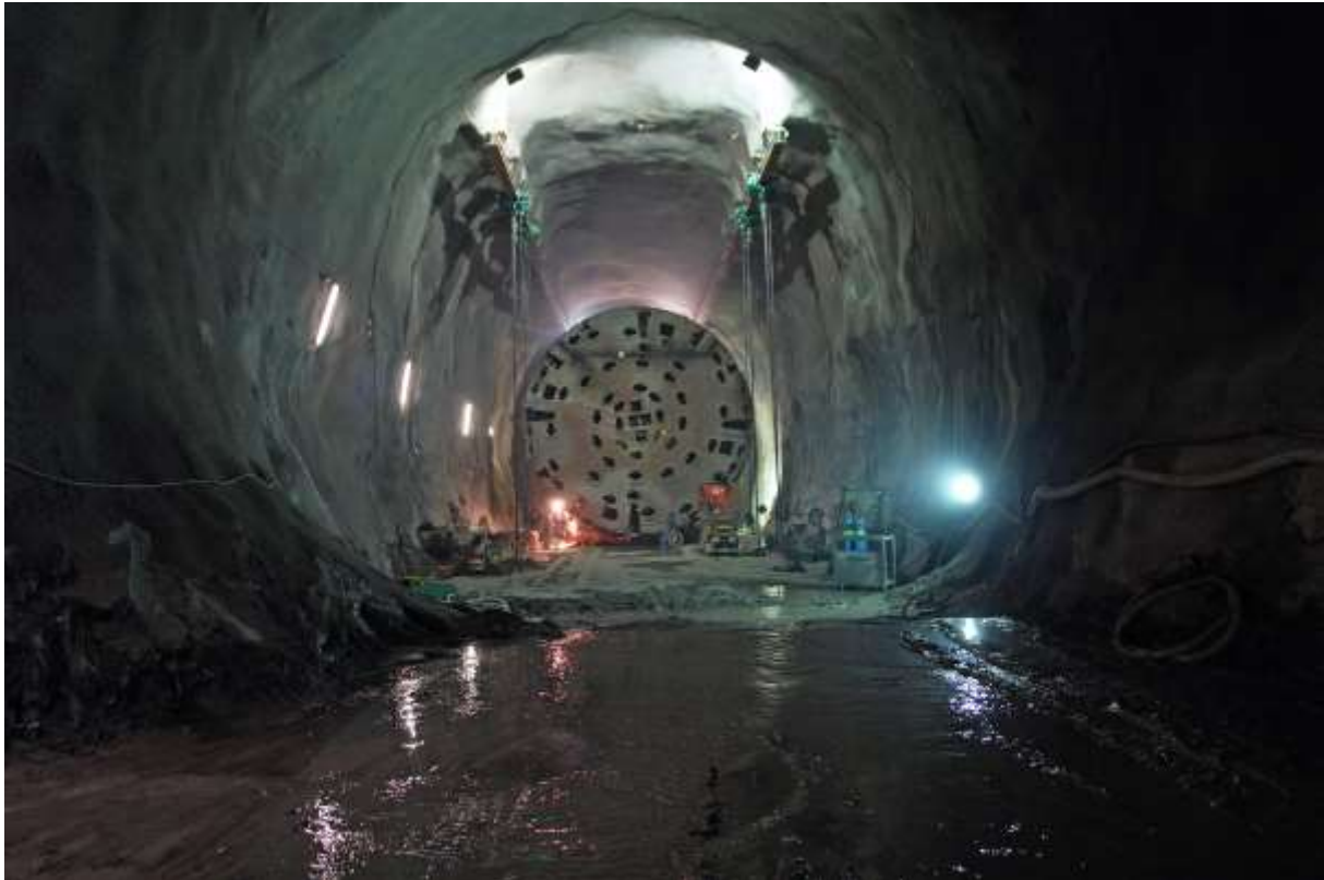
Copyright Alp Transit Gotthard AG, Sedrun Oströhre
