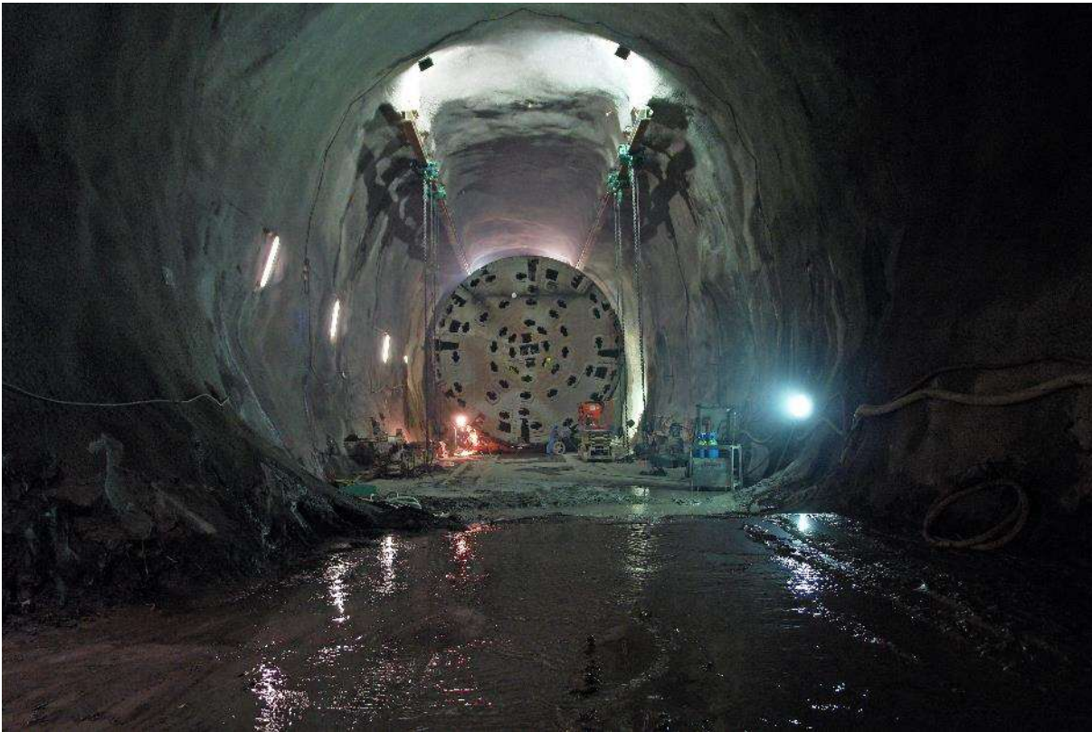
Copyright Alp Transit Gotthard AG, Sedrun eastern tunnel
