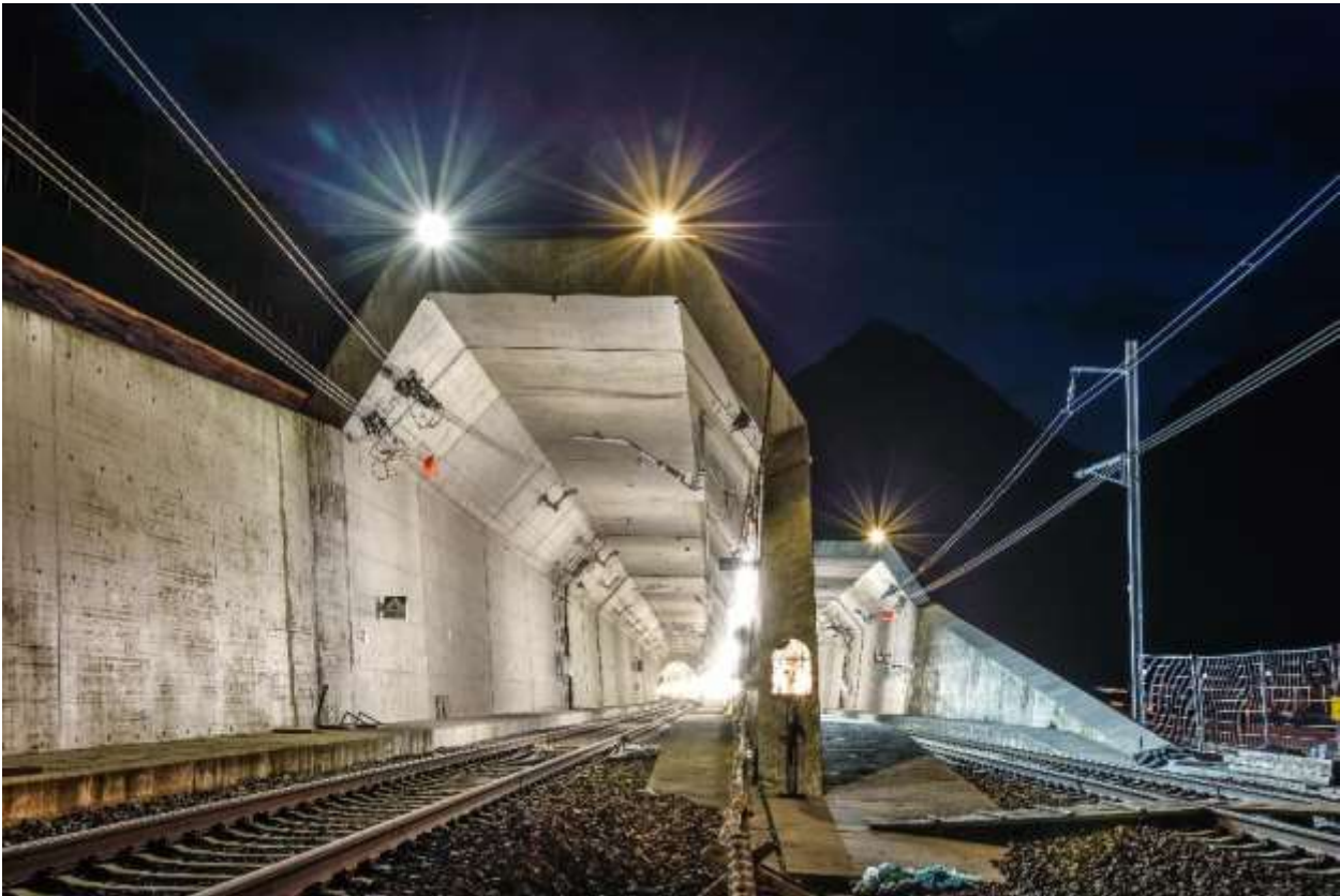
Copyright AlpTransit Gotthard Ltd, North Portal Erstfeld Gotthard Base Tunnel
