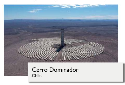
heat to a heat exchanger. There, the heat is used to heat a water stream which generates very hot steam. This steam powers a turbine which can generate more than 100 MW of environmentally friendly power. Thanks to the thermal storage, the power supply can be guaranteed 24 hours a day.
